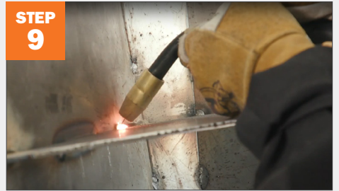
Weld the seat to the inside of the wings.
