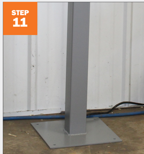
STEP 11 Mount base plate to floor with four bolts.
